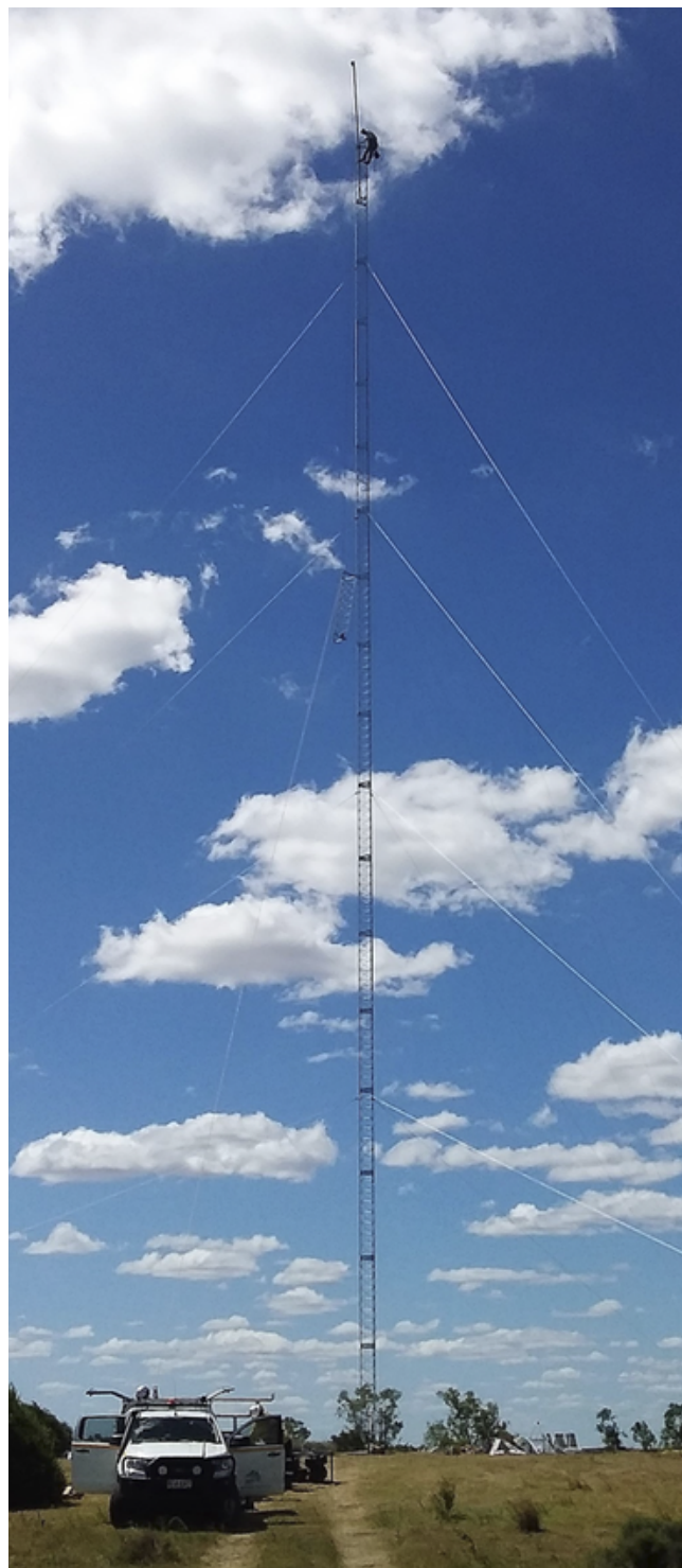
Figure 1: A Typical Meteorological Mast
