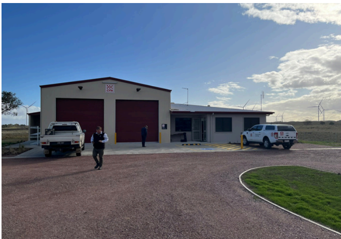
Photograph of the new CFA Shed (outside)
