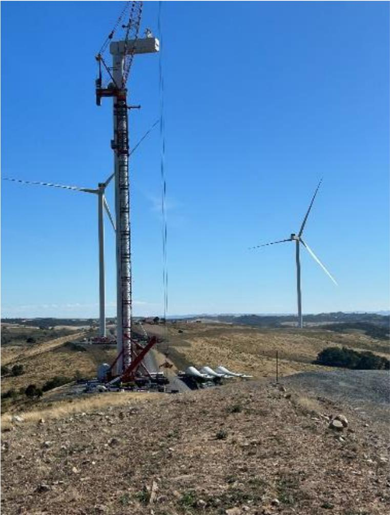
Photo 17: Turbine delivery and erection
