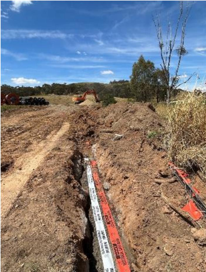
Photo 22: Cable trench backfilling
