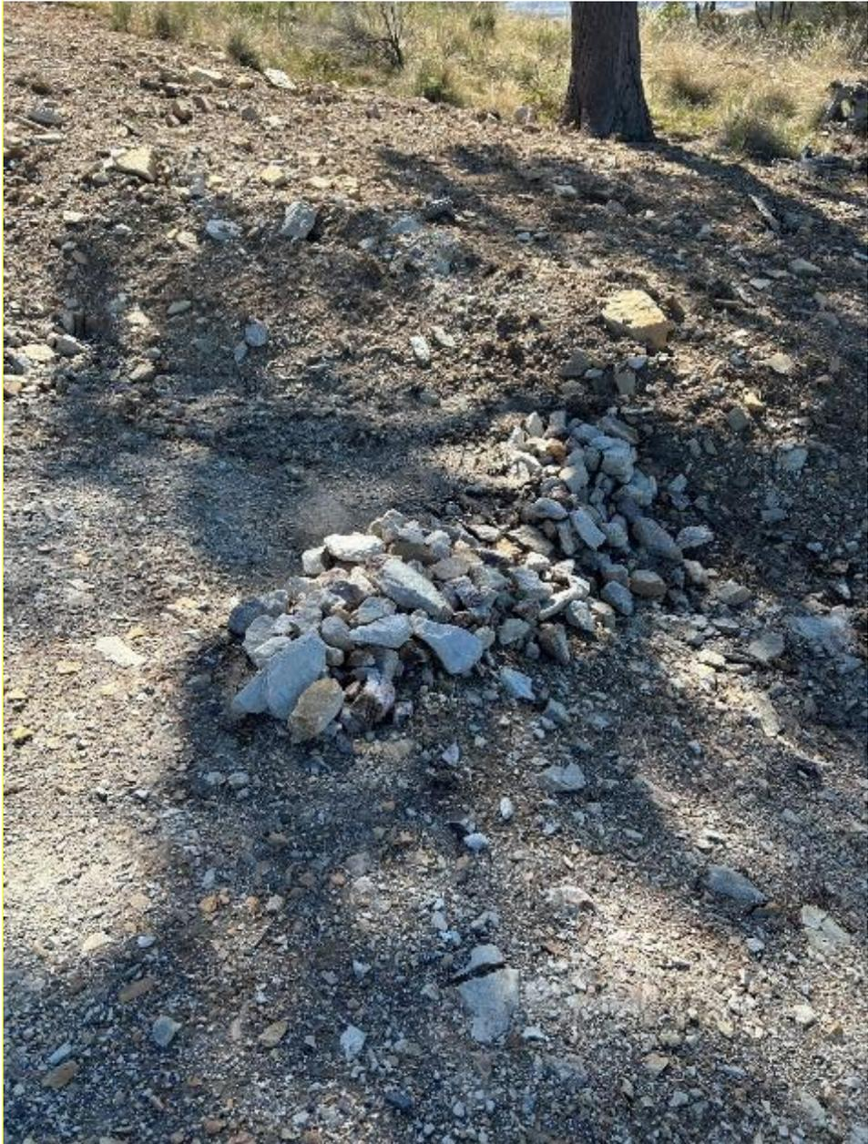
Photo 1: Road drain with rock check dam silted up and ineffective
