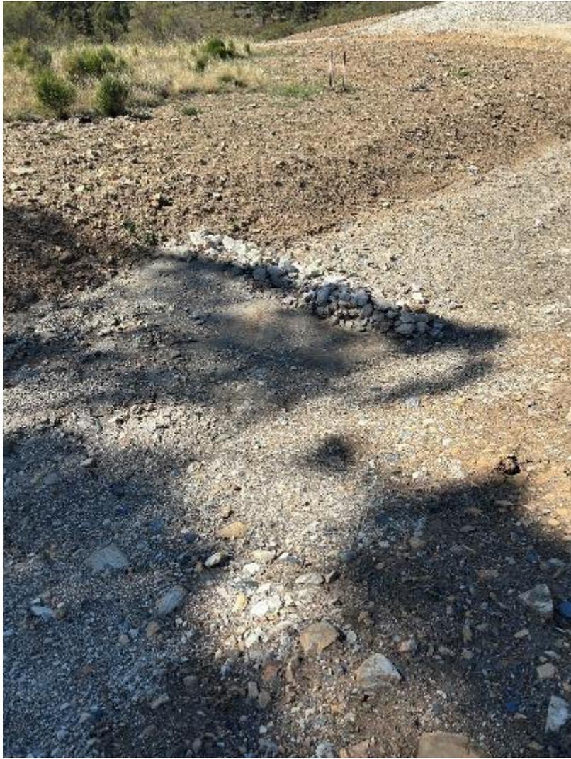
Photo 2: Road drain with rock check dam partly silted up and breached and ineffective.
