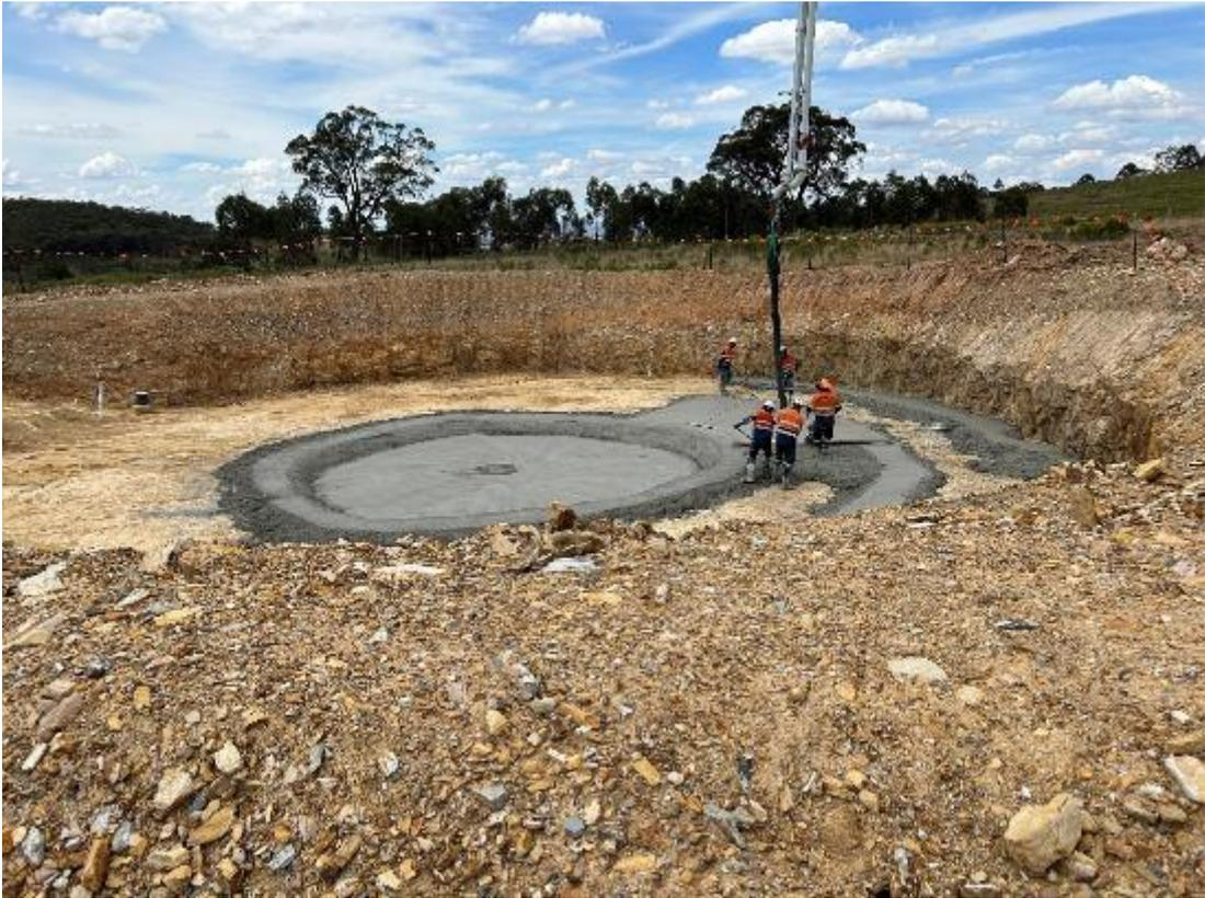
Photo 21: Footing concreting
