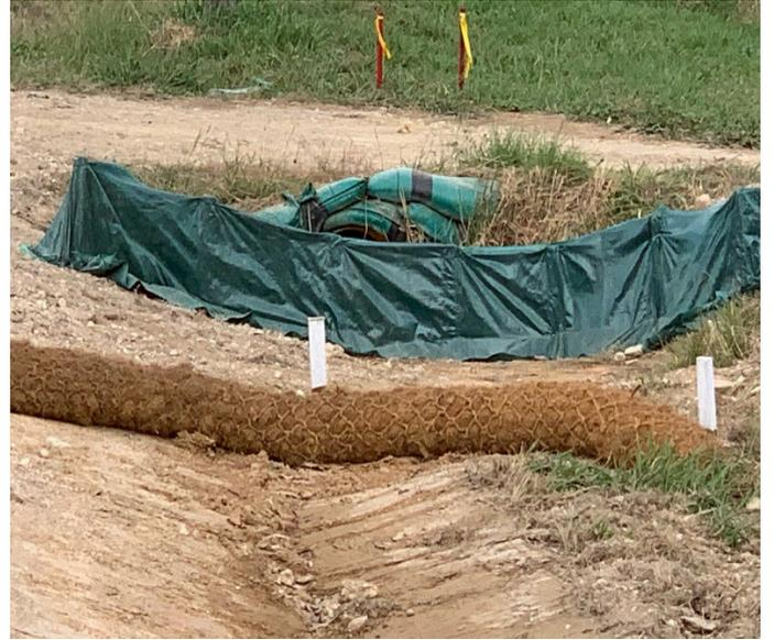
**Photo 6:** Erosion and Sediment Control, drainage protection
