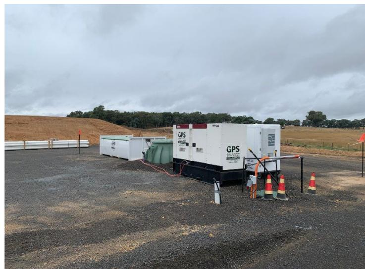
**Photo 12:** Double skinned fuel tank on hardstand area
