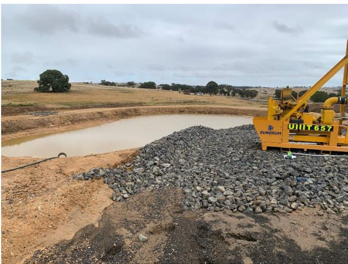
**Photo 11:** Sediment basin (water re-used for dust suppression)
