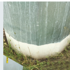
A pole directly embedded into the ground.
