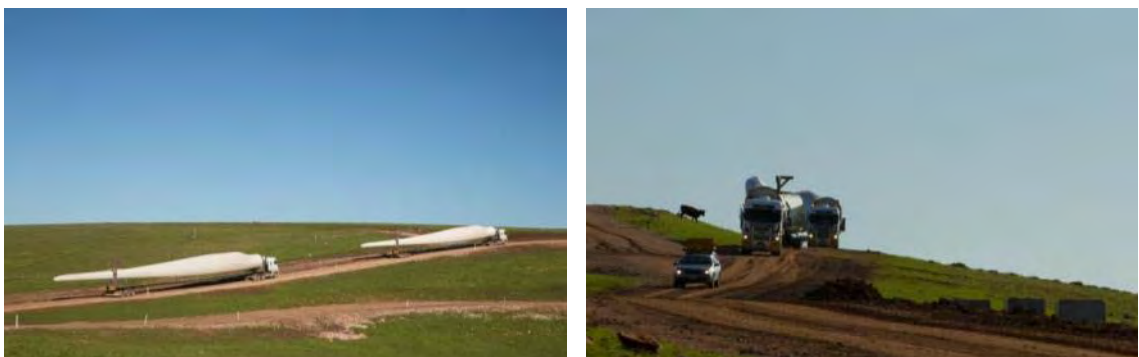
Figure 2 Examples of turbine parts being transported on site
