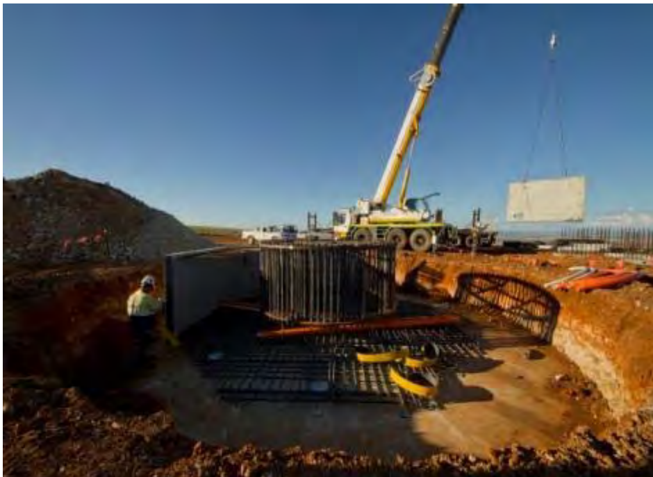
Figure 5 Example – construction of a turbine foundation/footing
