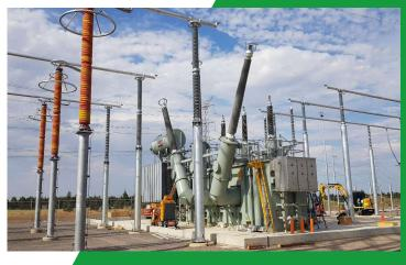
220/500kV main transformer installed
