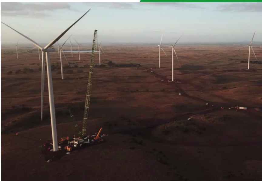
Turbine Install at F07
