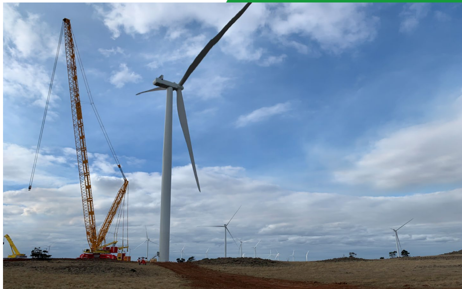
WTG installation at F05
