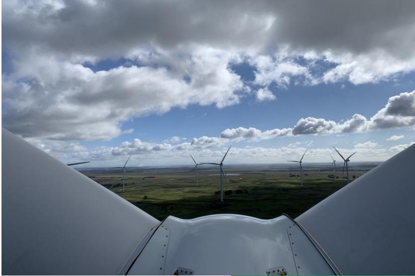
Views from the turbine-tops
