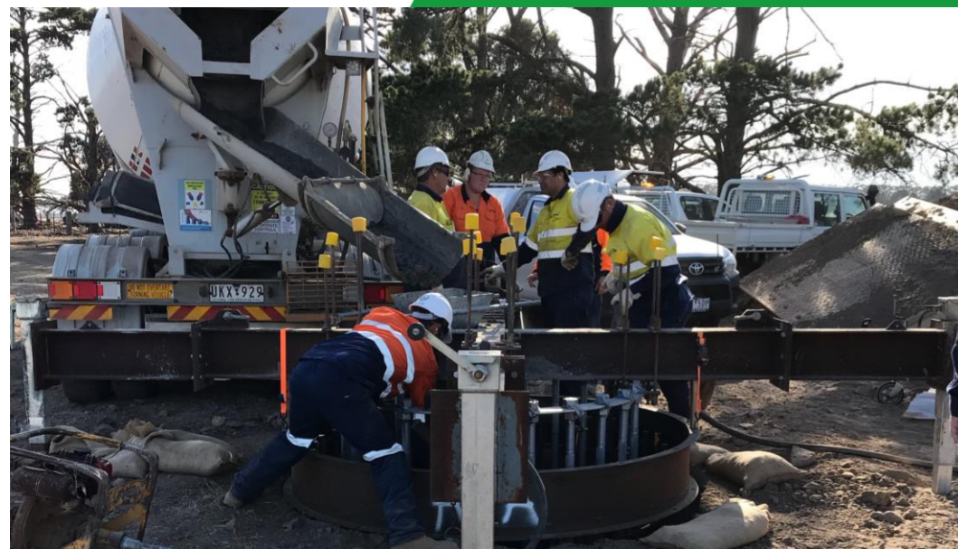
Pouring of transmission pole foundations
