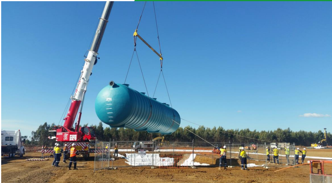
Settling tank being installed at the Blue Gums Substation
