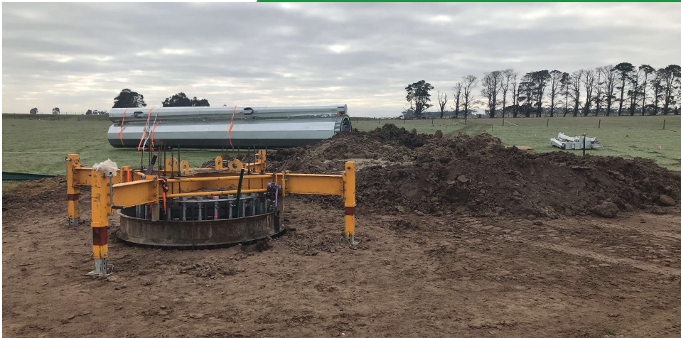
Transmission pole foundation set, and pole section delivered
