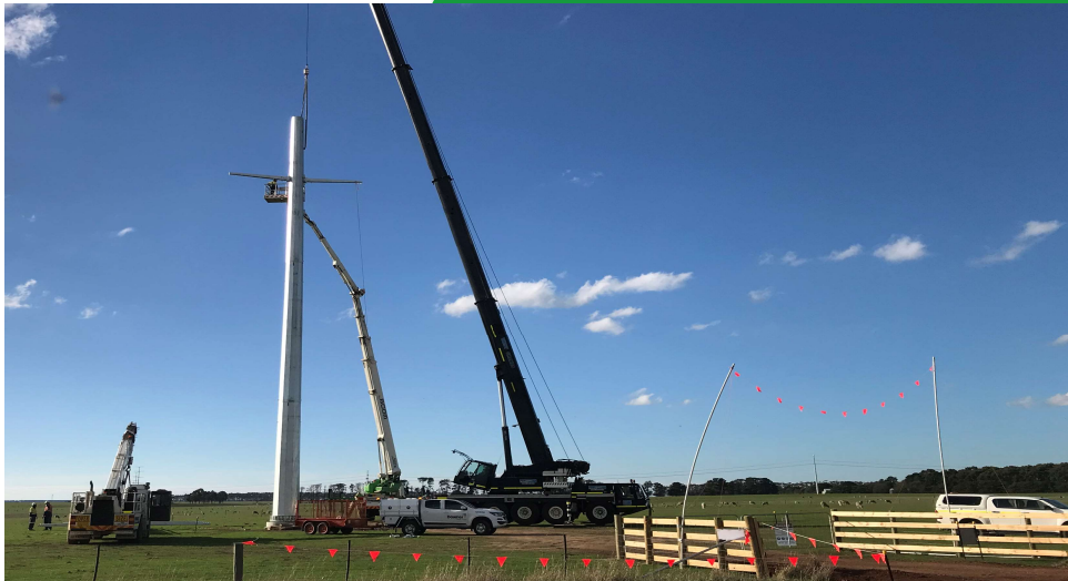
Assembly of a transmission line pole
