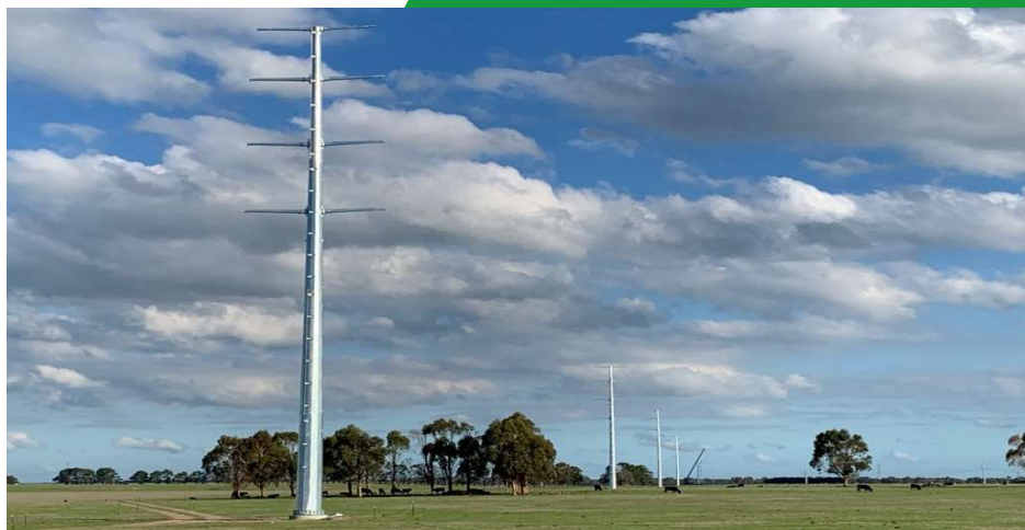
12 transmission poles now assembled
