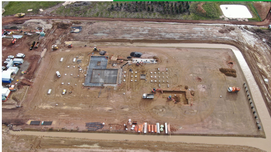
Blue Gums Substation progress
