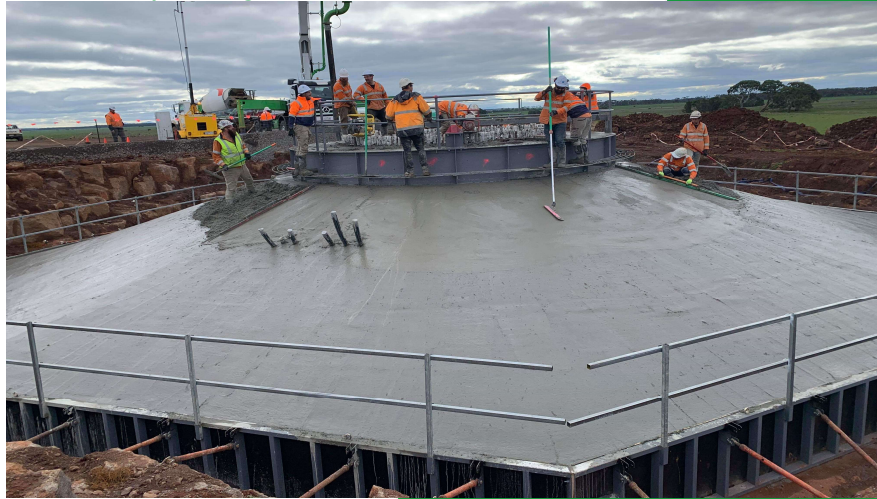
Concrete pouring of the first turbine foundation
