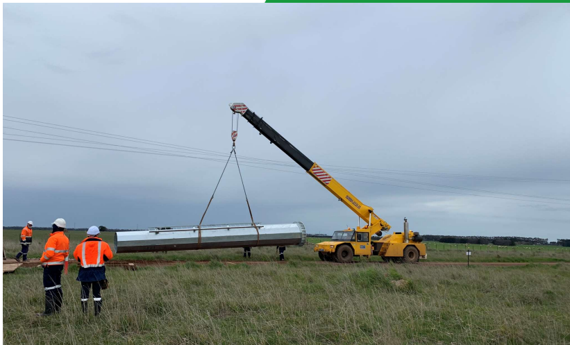
Transmission line pole section ready for lifting
