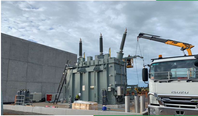
3-phase bushings installed on the transformer
