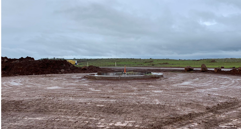
Foundation H02 Backfilled and Compacted
