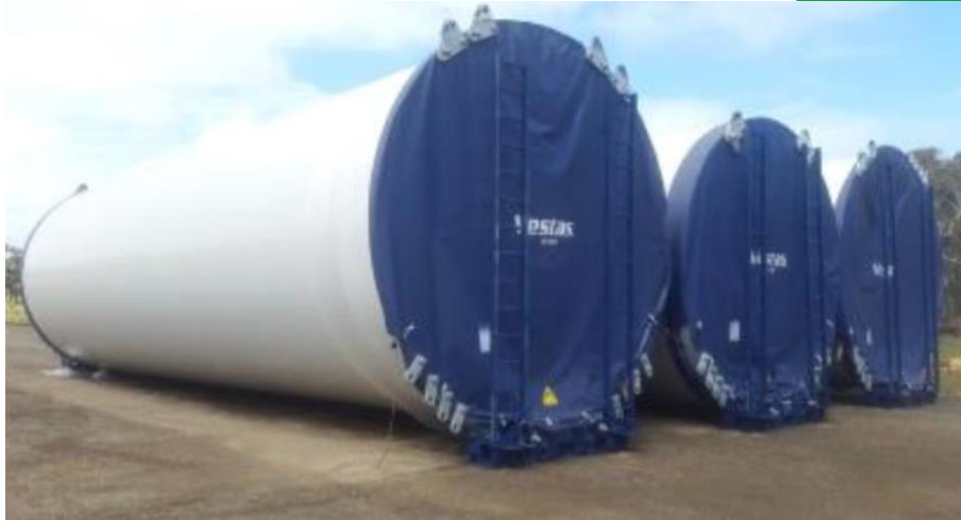
Arrival of wind turbine tower sections
