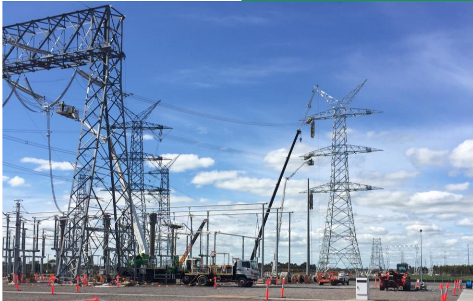
Tower construction and electrical works at MOPS
