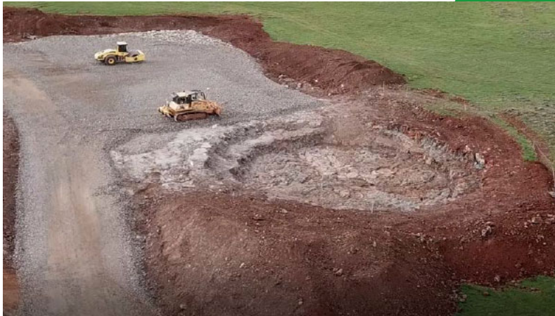
D01 hardstand and foundation construction
