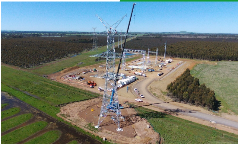
Stringing of optic fibre cable through tower 2
