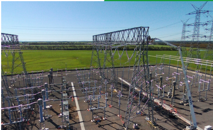
Connections works in MOPS switchyard
