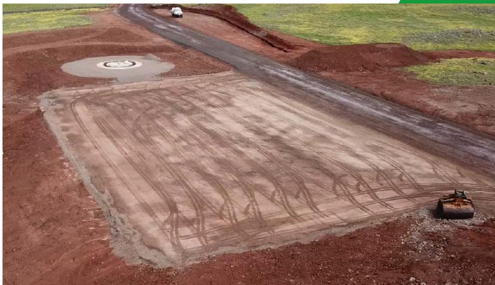
G05 foundation and hardstand civil works
