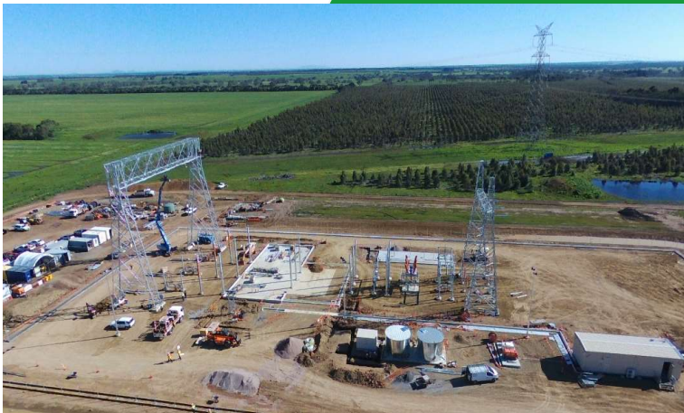
Blue Gums Substation progress
