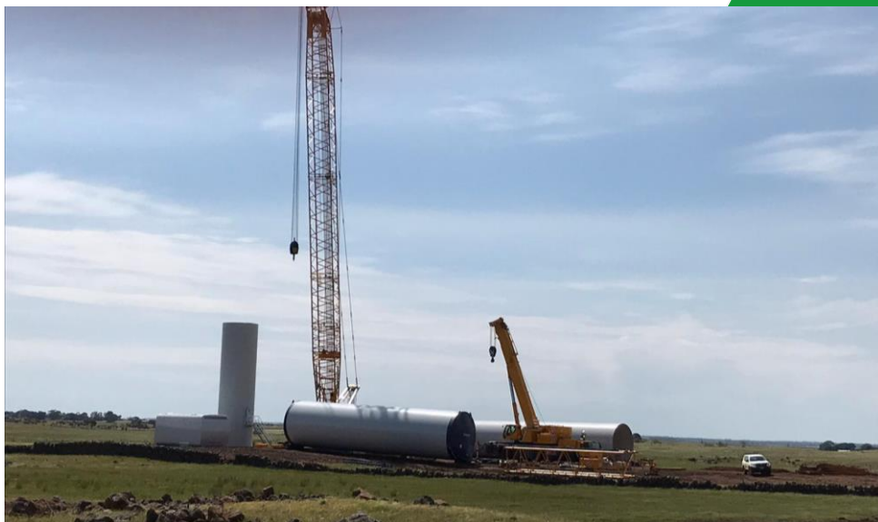
Standing of the first tower base section
