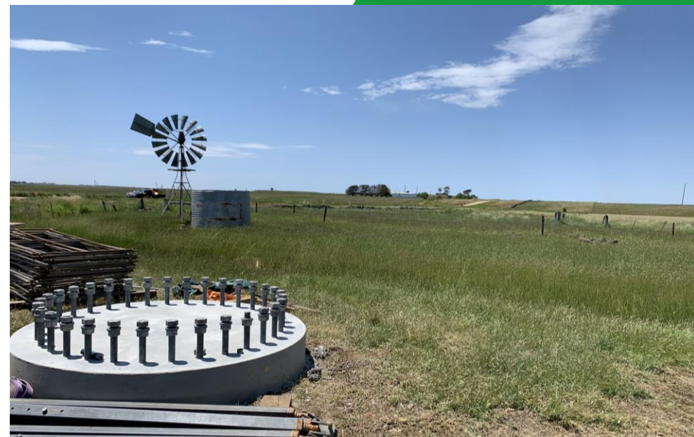
Transmission pole foundation construction
