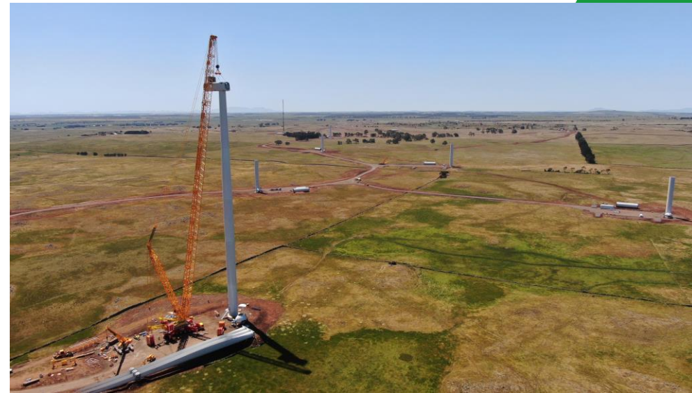
Main crane erecting wind turbine H09
