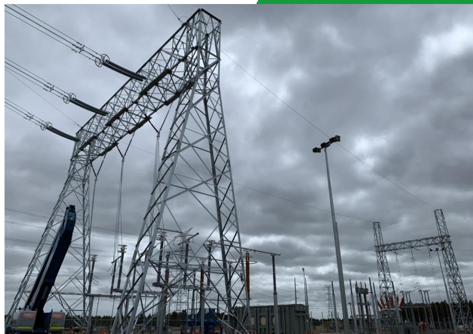
Stringing works at the Blue Gums Substation
