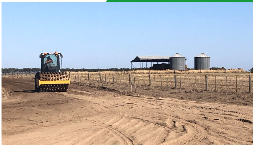
Stripping and compacting of the main access track
