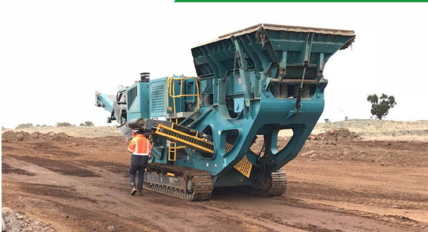
Rock crusher mobilising to the site compound
