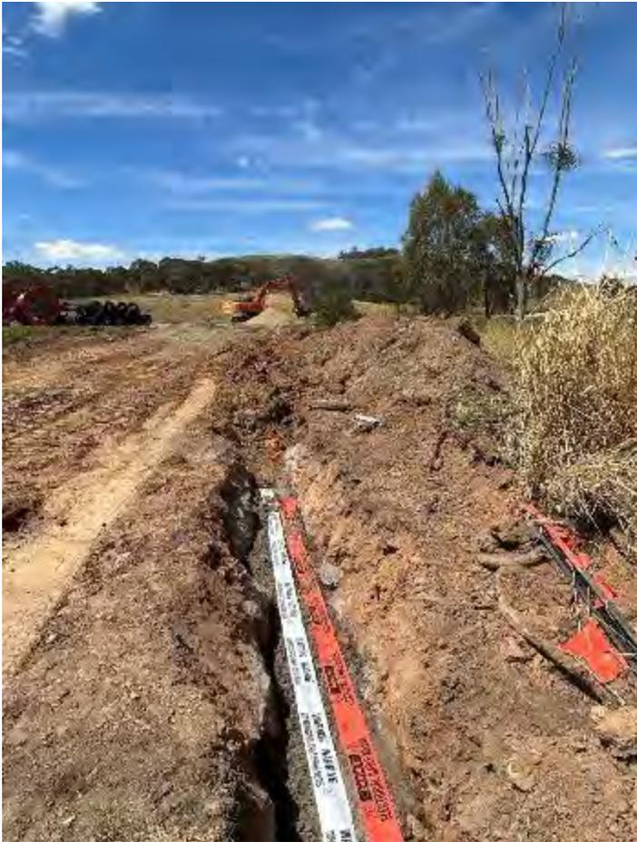
Photo 22: Cable trench backfilling
