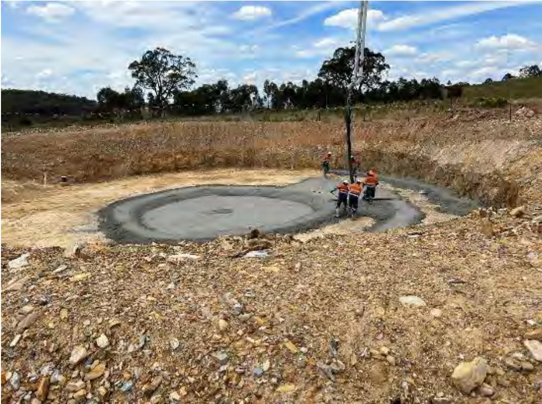
Photo 21: Footing concreting
