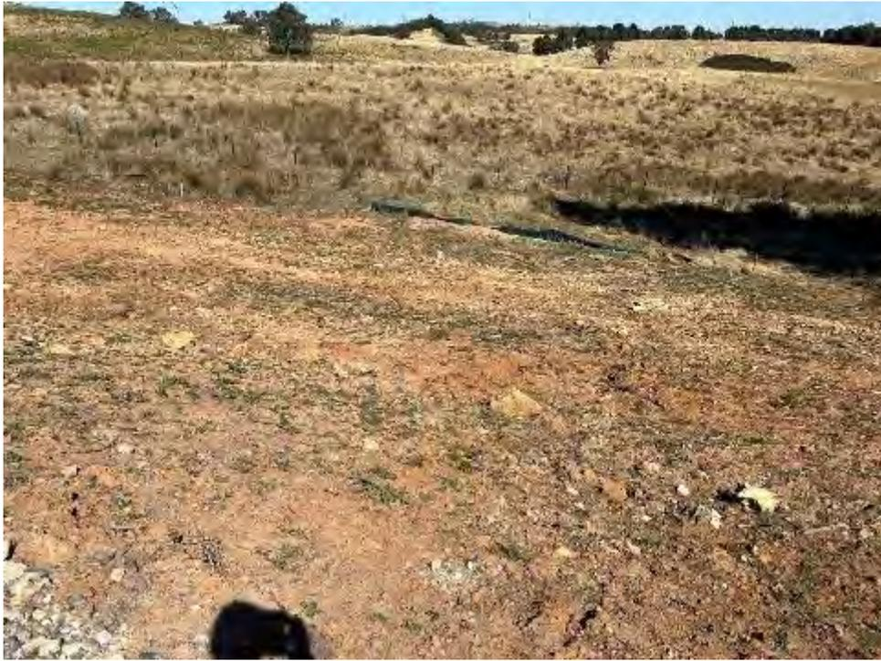
Photo 7: Sediment fence repair is required south of B11 where the cable run is eroding
