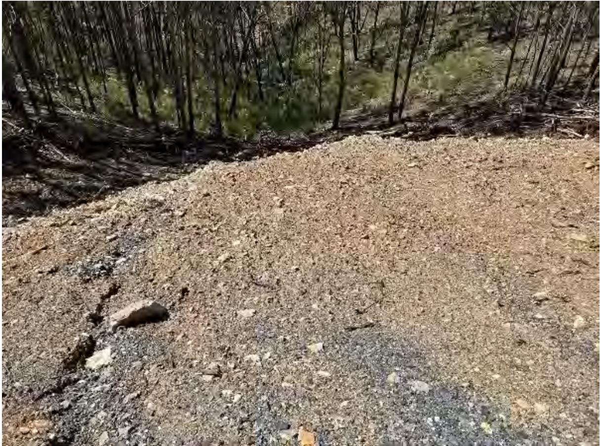
Photo 4: Embankment requiring stabilization at B15
