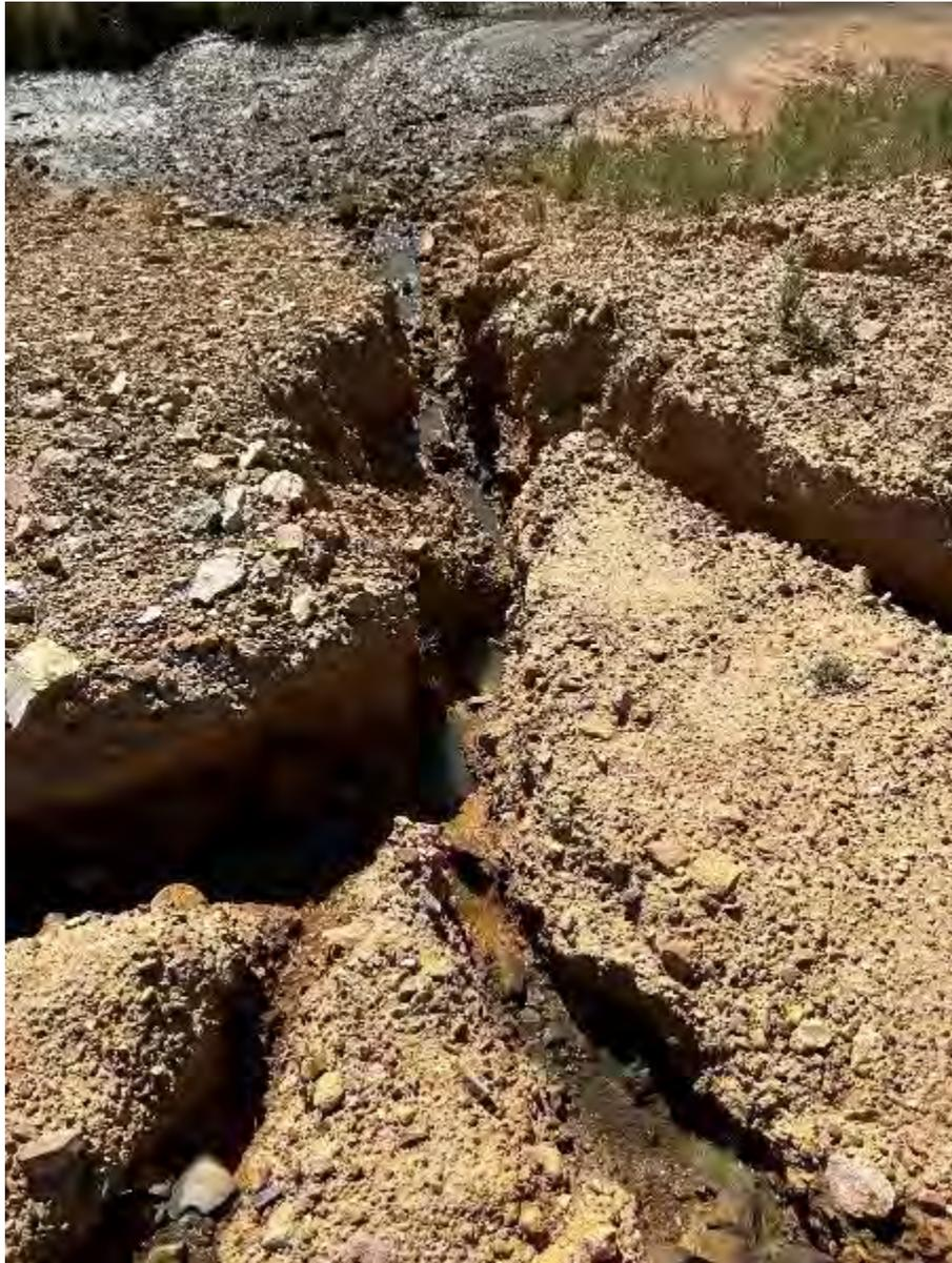
Photo 6: erosion caused by spillage from a standpipe at the northern batching plant (2)
