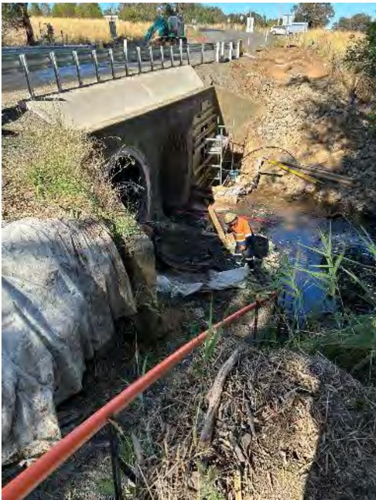
Photo 14: Environmental protection measures at Grassy Creek Road culvert relining
