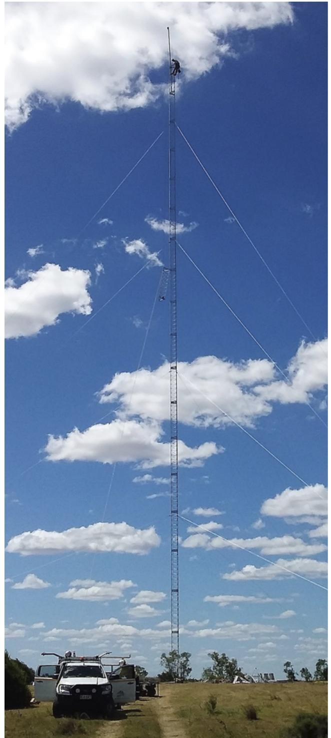
Figure 1: A Typical Meteorological Mast
