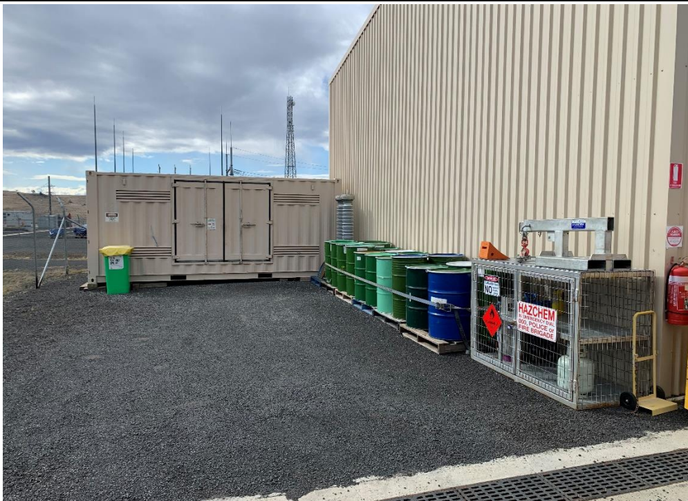
Photo 7: Empty containers stored neatly on pallets on hard stand for collection, Bunded and ventilated chemical storage container
