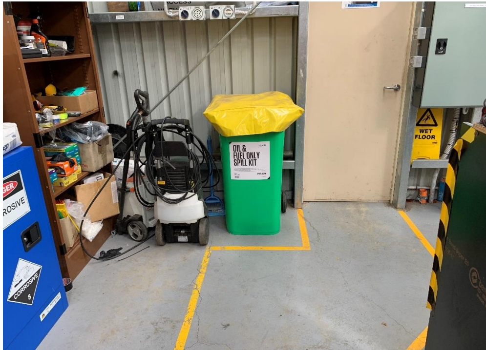
Photo 6: Spill kit and chemical storage area
