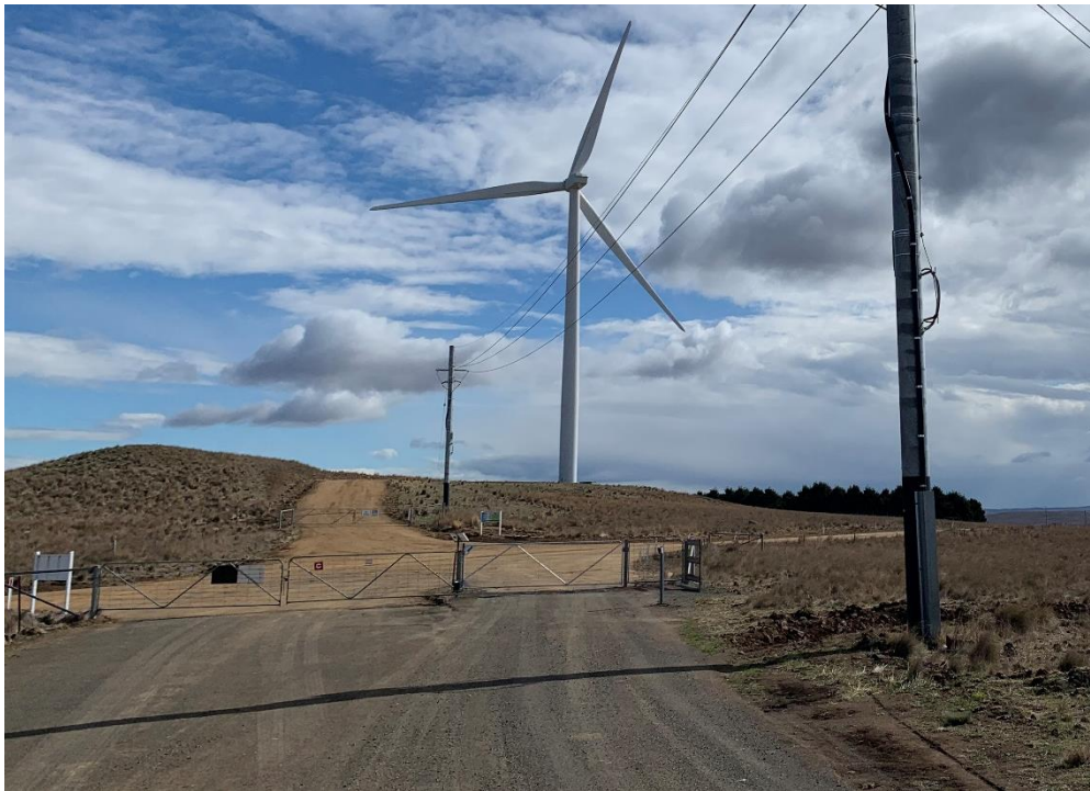
Photo 1: Avon Lake Road site entry. Stabilised site access and rumble grid to prevent mud tracking
